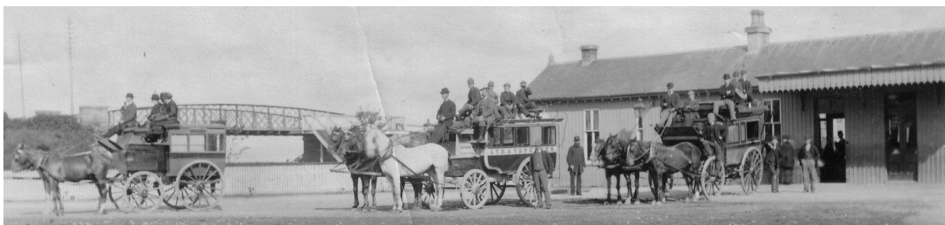
Dingwall's first station, before the rebuilding of 1886. Photo: Dingwall Museum
