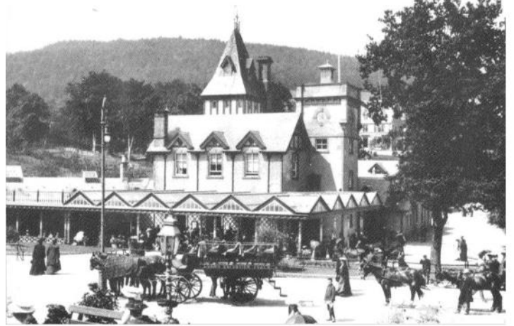
The Lower Pump Room, before 1910. Photo ©Margaret Spark
